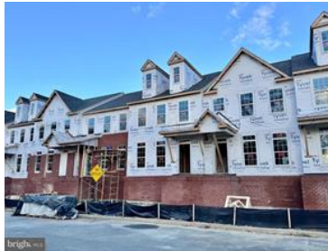
Currently under construction
