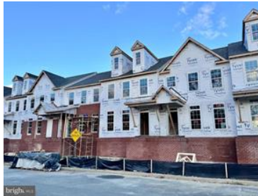
Currently under construction
