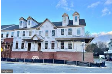
Interior unit pictured third from right
